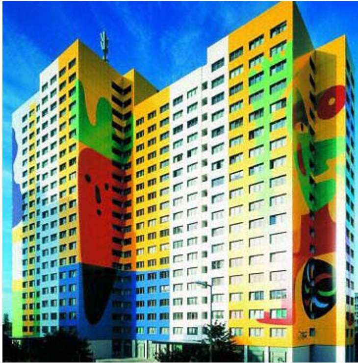
Picture 7: Berlin (renovation of old building)
