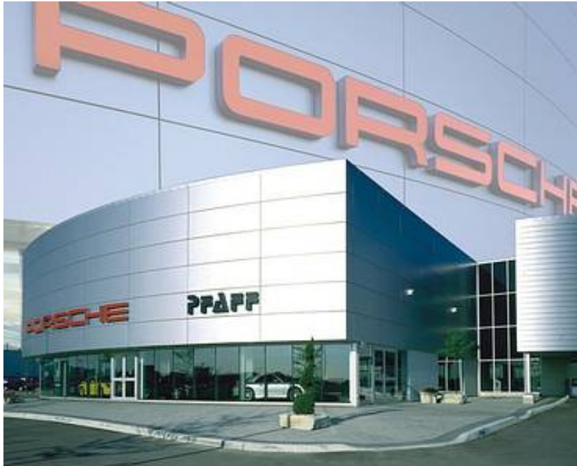
Picture 2: One of the first projects with ACP
